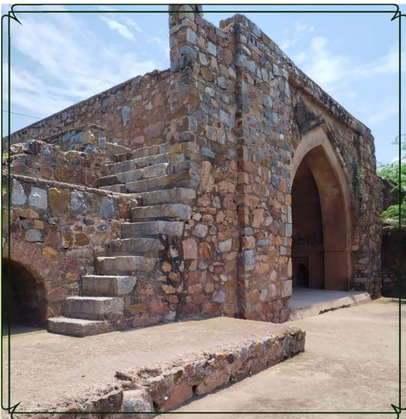
Outside View of Watch Tower
